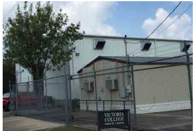
VICTORIA COLLEGE LIBERTY STREET INDUSTRIAL TRAINING CENTER 1404 N. Liberty, Victoria, TX 77901
