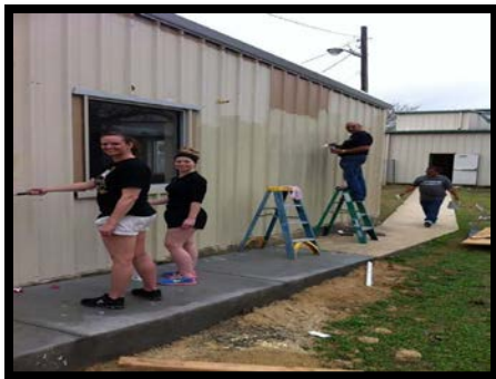
VC students help paint the newly renovated YMCA building.
